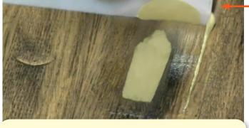
HINT: Fill all daylight gaps with KEY Polymer CrackFiller. When completed, use any excess CrackFiller to fill gouges in the wood.
